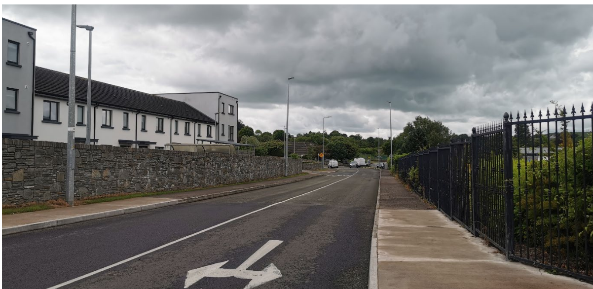
Plate 1.5.9 View westward along Mechterstadt Road
