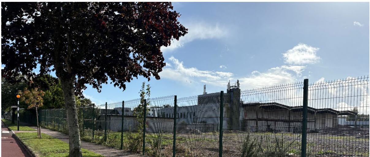
Plate 1.5.5 View southward from Innishmore Lawn showing northern boundary of site and adjoining site.
